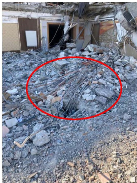
Ground floor column ore and reinforcements
